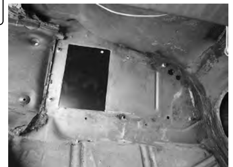
OEM Insulation Removed
